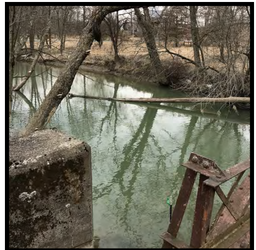
CC-1 Downstream View
